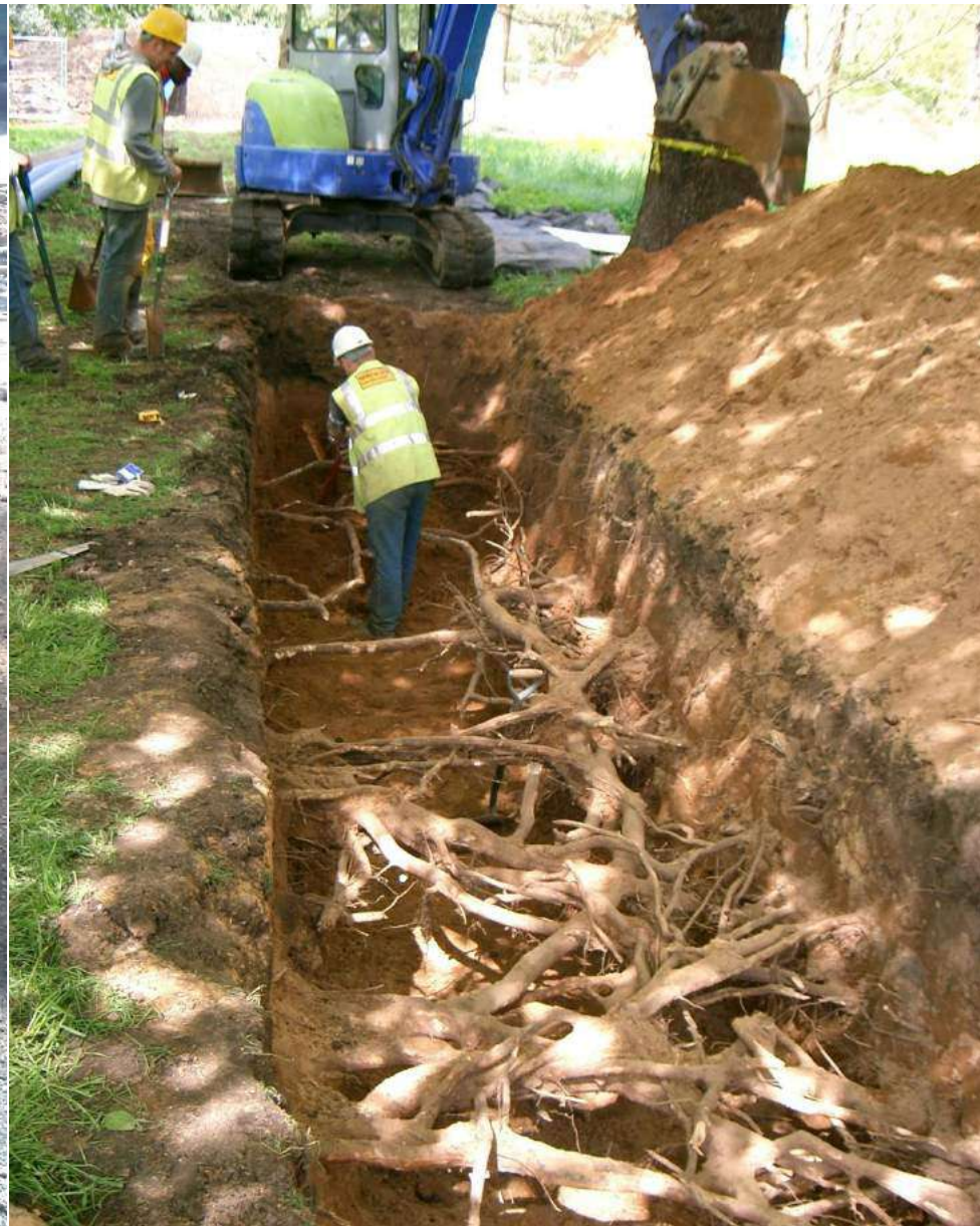
Excavation by hand, air spade and mini digger
