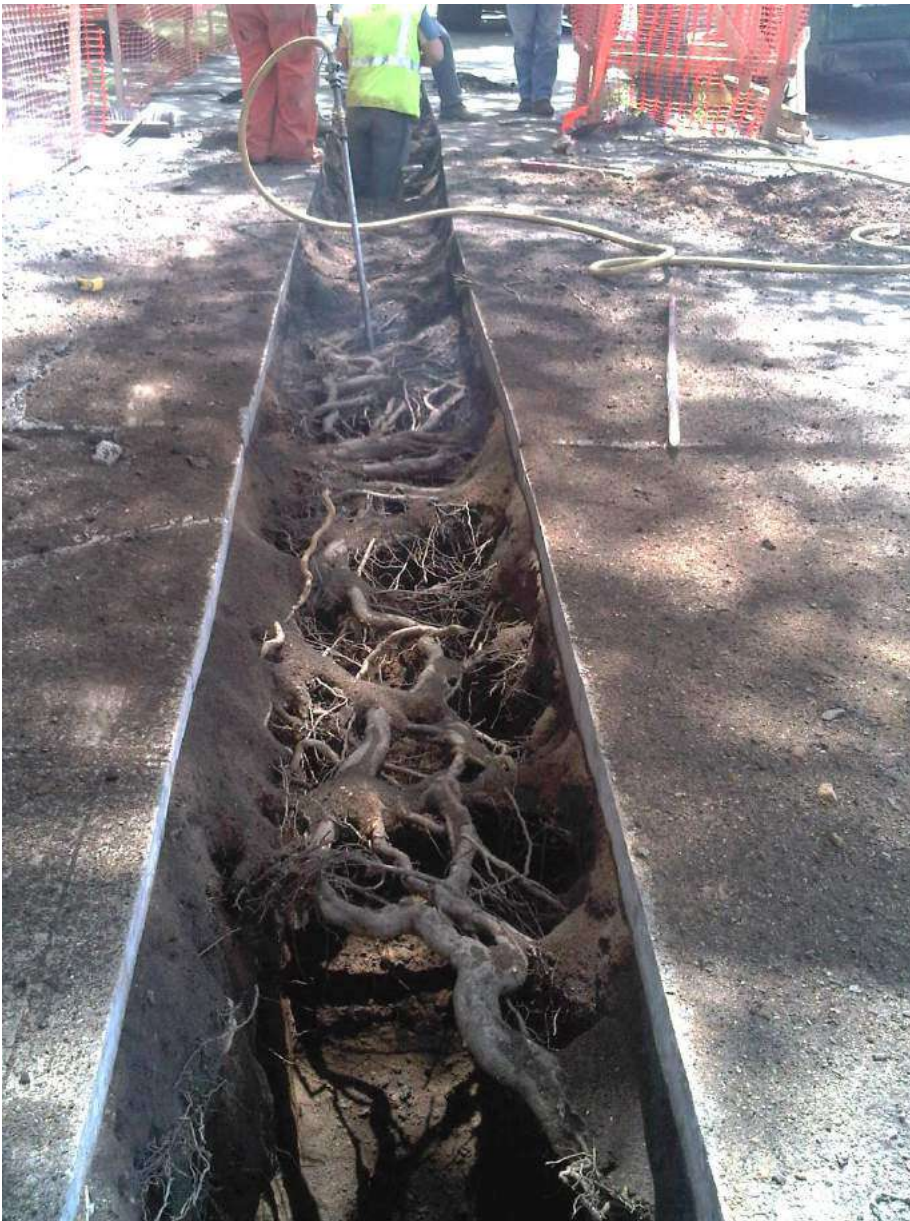
Excavation using an air spade
