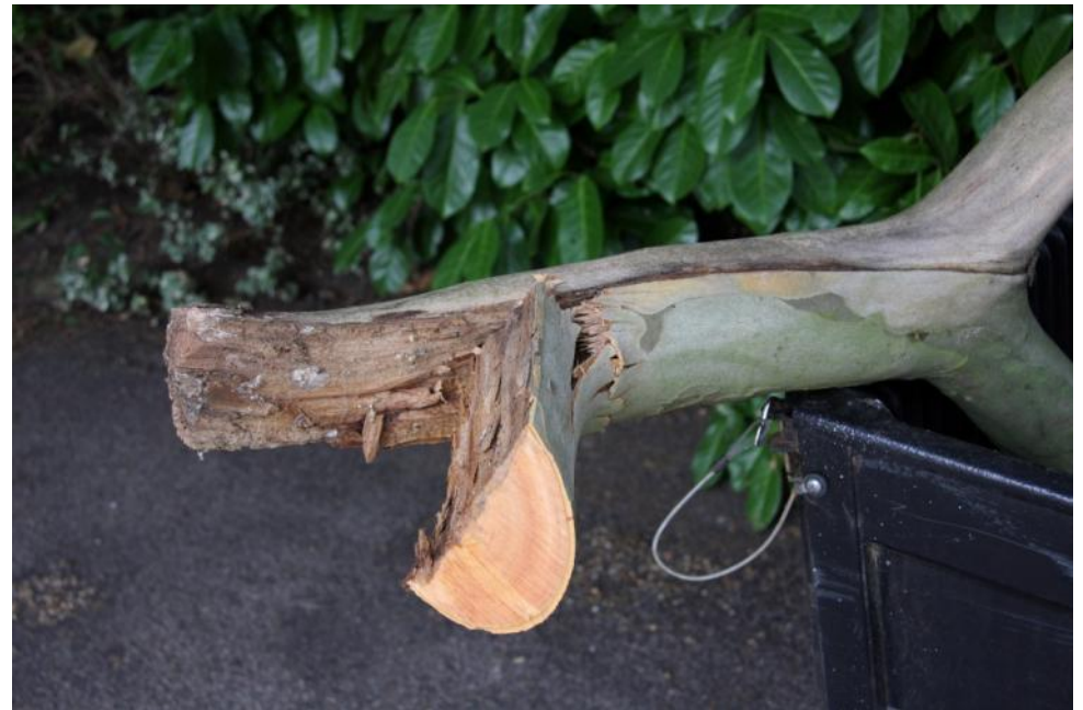
Failed Massaria limb from the Broadwalk Hyde
