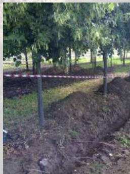
Trenching on 1 side of the tree - MD
