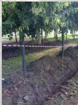
Trenching on 1 side of the tree - MD
