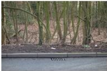
Monton Road, showing alignment of highway drains and existing woodland.
