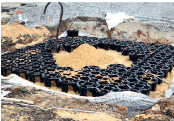
Installation of engineered solution in St Peter's Square, Manchester
