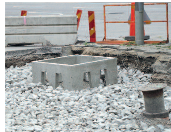
Installation of the Stockholm Structural Soil System
